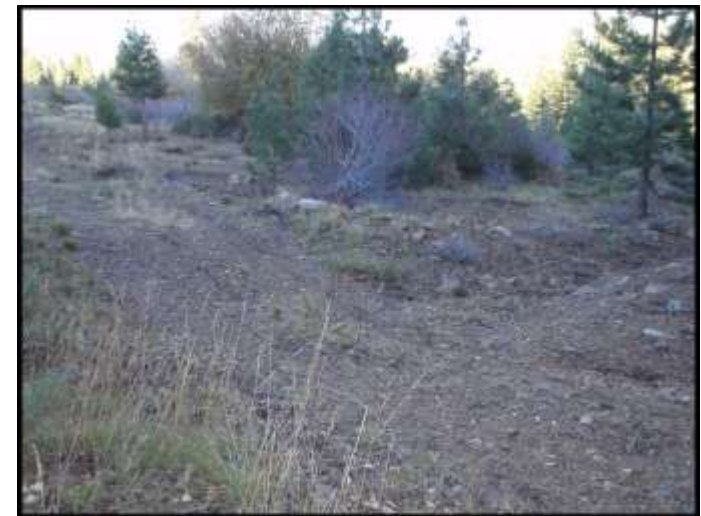
Photo 10d – Typical Existing Rolling Dip Needing Improvement
