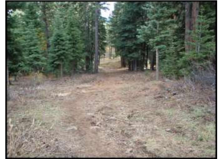
Photo 12a – Upper Reach of Project Typical of Rolling Dip Improvement
