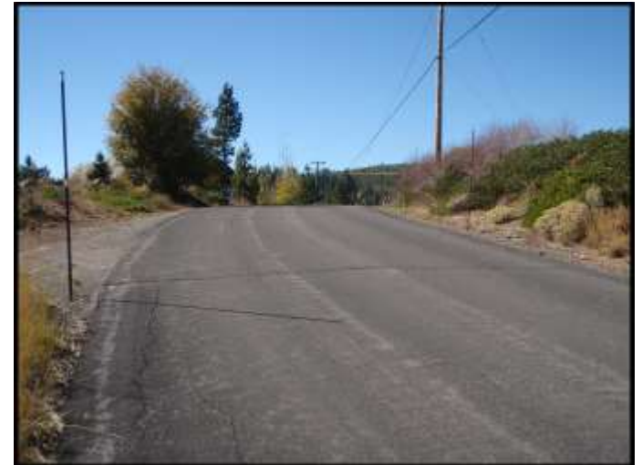
Photo 13b – Location of Project Crossing of Skislope Way
