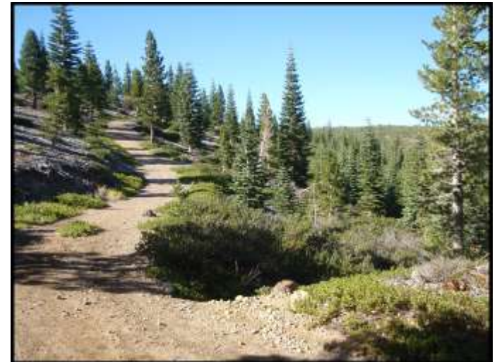
Photo 14b – Section of Existing Dirt Road and Culvert Utilized for +/- 30' of Trail
