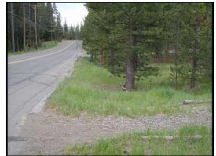
Photo 21b – Existing Clubhouse Trail North of Lausanne Way Intersection Looking West
