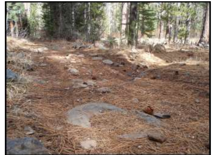
Photo 22d – Typical Existing Rolling Dip Condition of Segment 22D Proposed for Improvement
