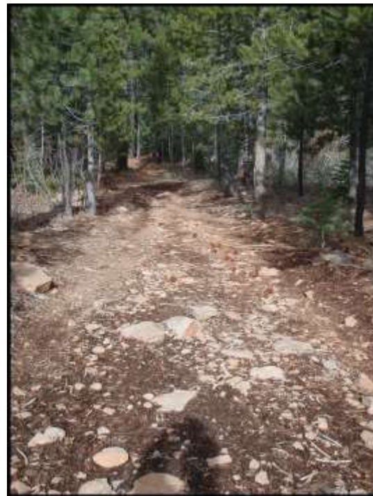
Photo 22e – Typical Fall Line Erosion Condition of Segment 22D
