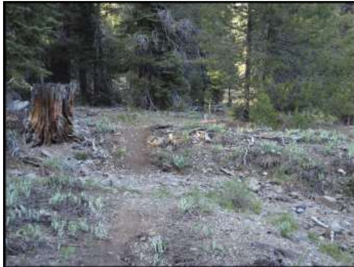
Photo 3e – Trail Crossing of Large (<20 cfs design flow) Drainage Path w/ Rock Lined Rolling Dip
