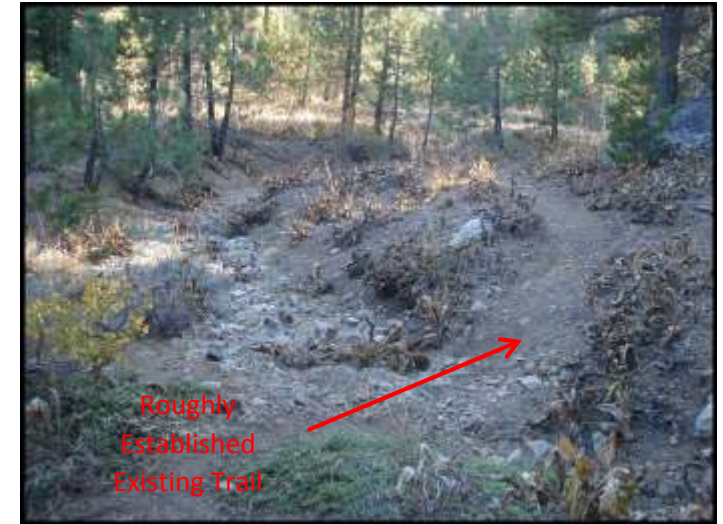
Photo 3c – Trail Crossing of Medium (<5 cfs design flow) Drainage Path w/ Rock Lined Rolling dip
