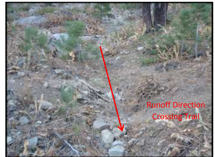
Photo 3b – Typical Trail Crossing of Small (<2 cfs design flow) Drainage Path
