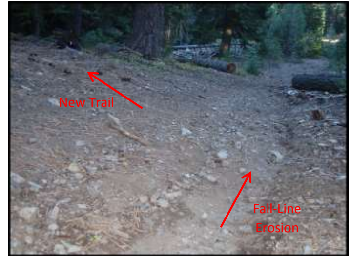
Photo 4a – Existing Road (Lower / East Segment) Erosion at New Trail Intersect
