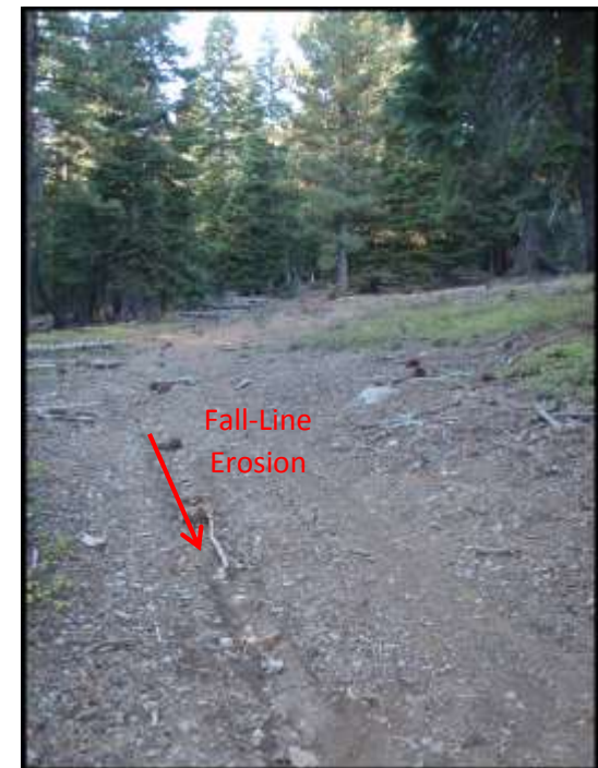
Photo 4b – Existing Road (Upper/West Segment) Fall-Line
